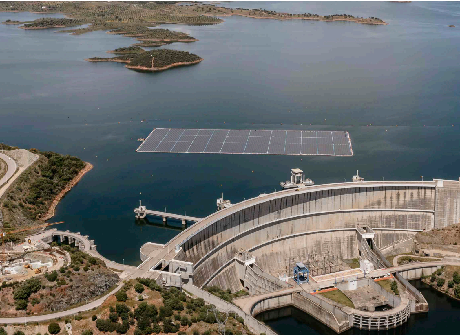
FIG. 3 FLOATING PHOTOVOLTAICS, ALQUEVA
