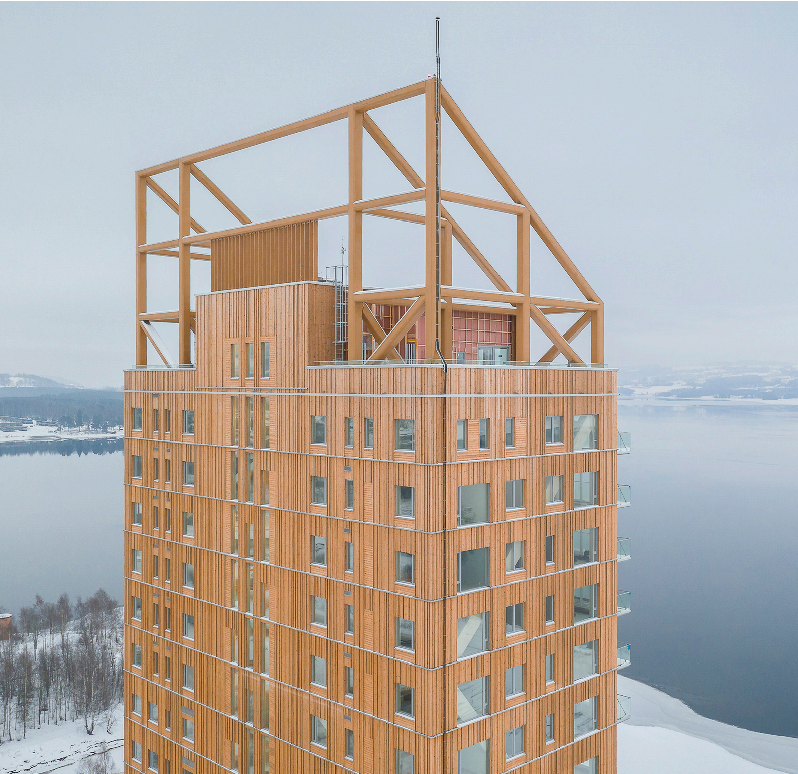
FIG. 8 18-STORY BUILDING IN NORWAY, MADE ENTIRELY FROM WOOD
